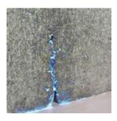
Photograph shows a crack in a block wall before the seam tape is applied.
